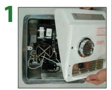
Remove your existing dryer, leaving the electrical box in place.
