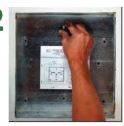
Insert COLUMBIA VORTEX electrical box with provided fasteners.
